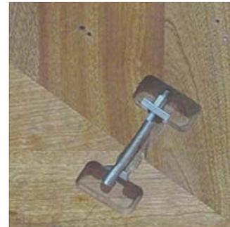
Joints are secured with T-Bolt hardware installed on the underside of the countertop.
